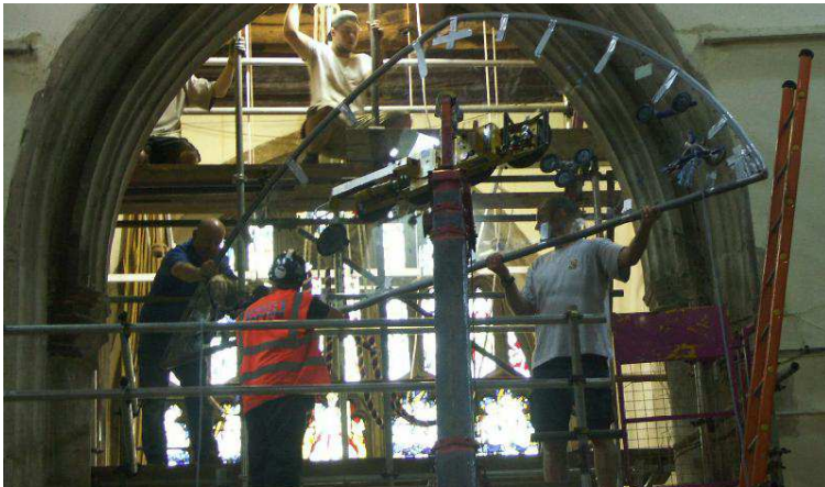
Guiding the glass through the arch The new base unit below the glass
