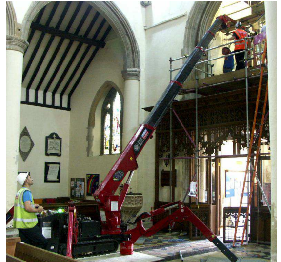
Crane lifting the glass into place
