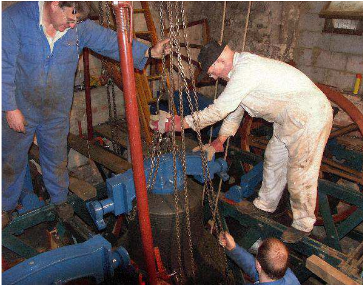
Lowering a bell into its pit
