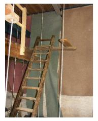
In 2005 the ringers hung old carpets on the walls of the clock room to reduce the internal reverberation and enhance the clarity of the bells as heard by the ringers below. This simple, cheap treatment proved very effective.
